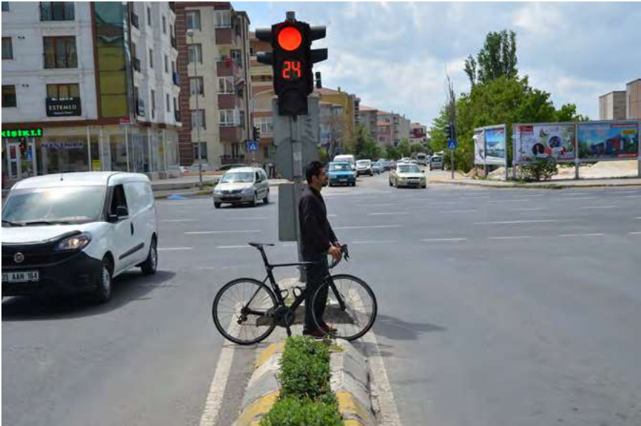
Pedestrian islands at traffic lights that are too small
